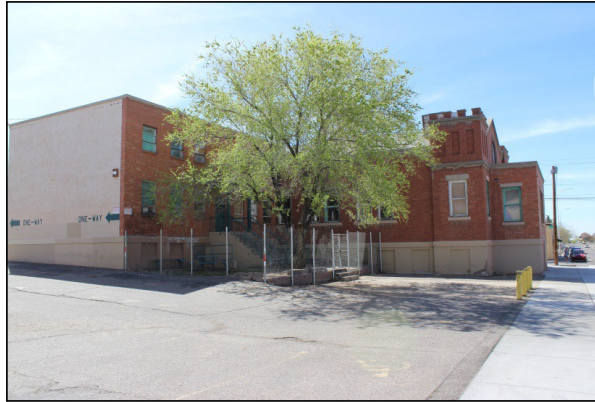
Vacant and deteriorating building fronting Broadway Blvd.
